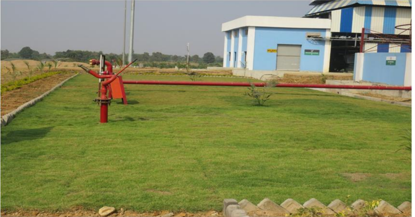
Annexure-III: Pictures of Rain Water Harvesting Structure
